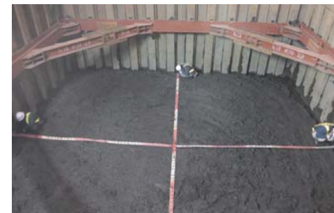
掘削完了確認
