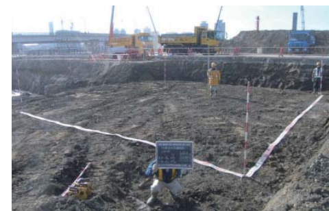
掘削完了確認
