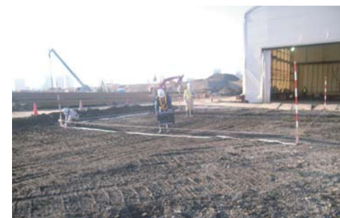
掘削完了確認
