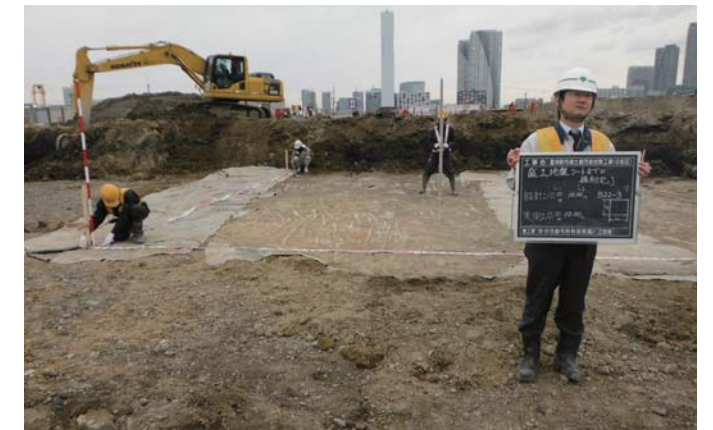
掘削完了確認
