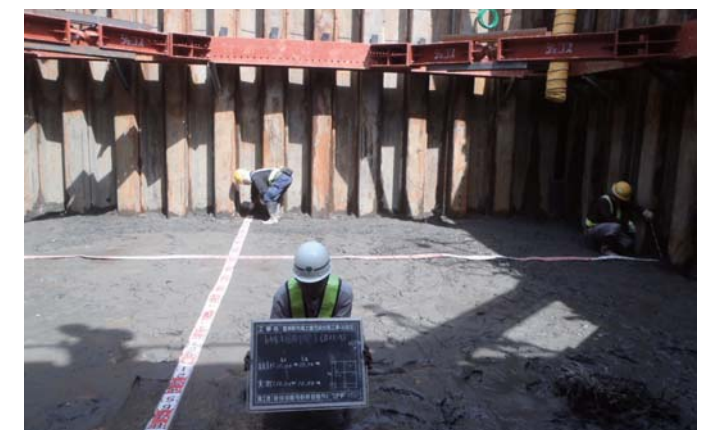
掘削完了確認
