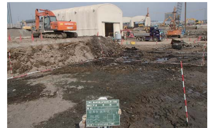
掘削完了確認
